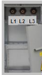
Figure 29 – Marking of the phases
