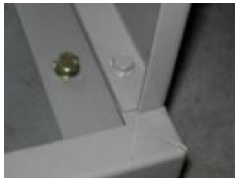
Figure 26 – Floor fixing example
