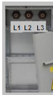
Figure 29 – Marking of the phases
