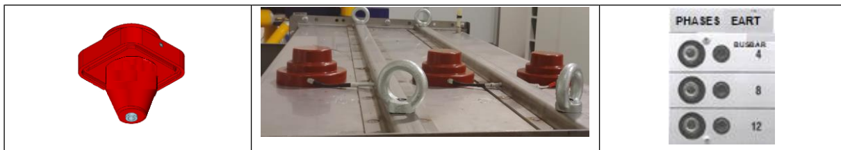
Figure 30 – Bushing of the capacitive voltage divider and connection of the busbar VDS (not bidding).
