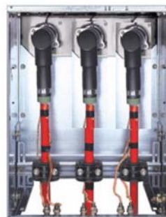
Figure 28 - Examples of Supports and Separable connectors installation
